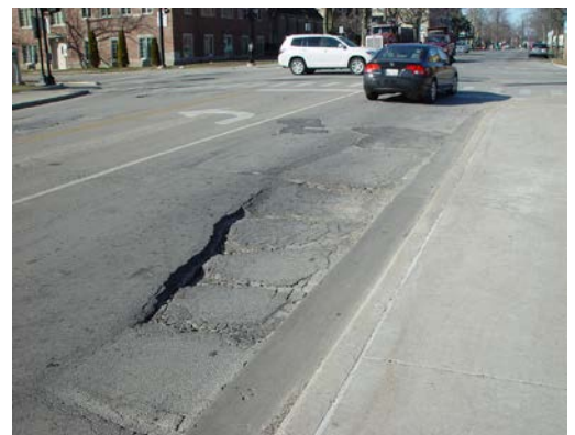
Wright Street Existing Pavement Condition
